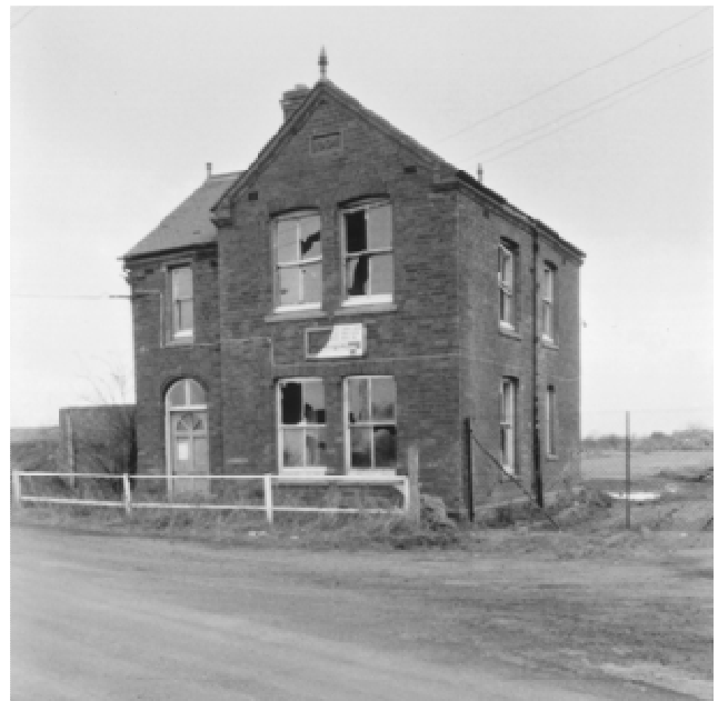
Brickyard Site Managers Building (built 1904)
